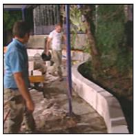
**Pathway:** Jamie drew on the concrete pathway the new shape and then with a wet saw, which we hired, proceeded to cut along the lines. Once the cuts were made we jackhammered out the areas for the garden beds. We used a quick drying paving paint to give us another dimension.
